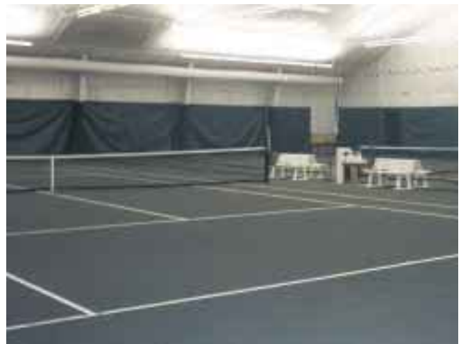
The Snowmass Club tennis center lighting system is one of the most efficient in the world.
